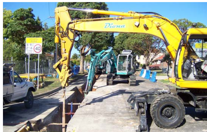
Lowering pipe into the trench
