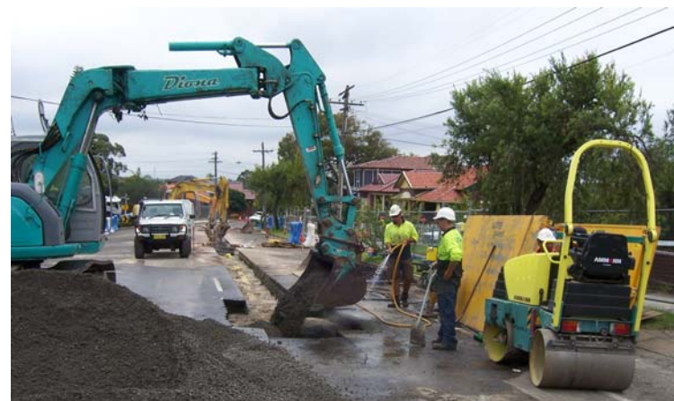
Commencing road pavement reconstruction
