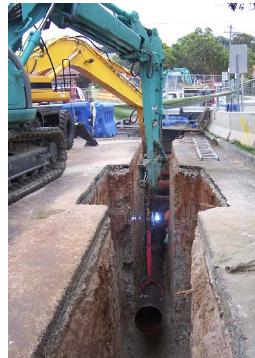
Welding similar pipe in the suburbs of Sydney
