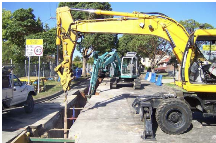
Lowering pipe into the trench
