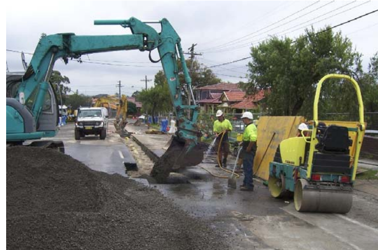
Commencing road pavement reconstruction
